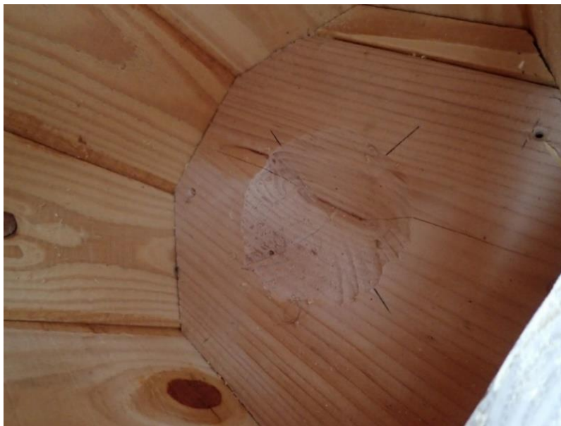
Inside floor of octagonal box with 4" diameter \frac{3}{4} " deep circular concave area cut in a 1.5" thick wood bottom, providing insurance in case starlings remove all bedding before kestrels take over box. A 6.5" circular saw blade works best for this cut, set at \frac{3}{4} " depth. The thicker bottom insulates eggs better.
